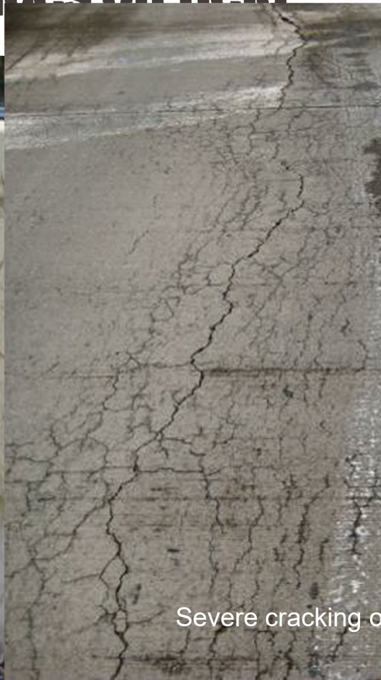
Important cracking on highway barrier wall
